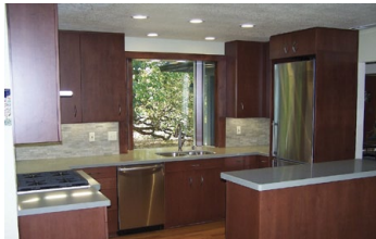
Labourdette Construction recently completed this kitchen remodeling project.
